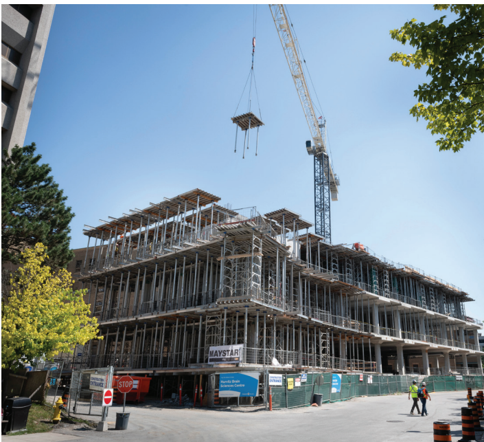
Garry Hurvitz Brain Sciences Centre, with construction underway.
